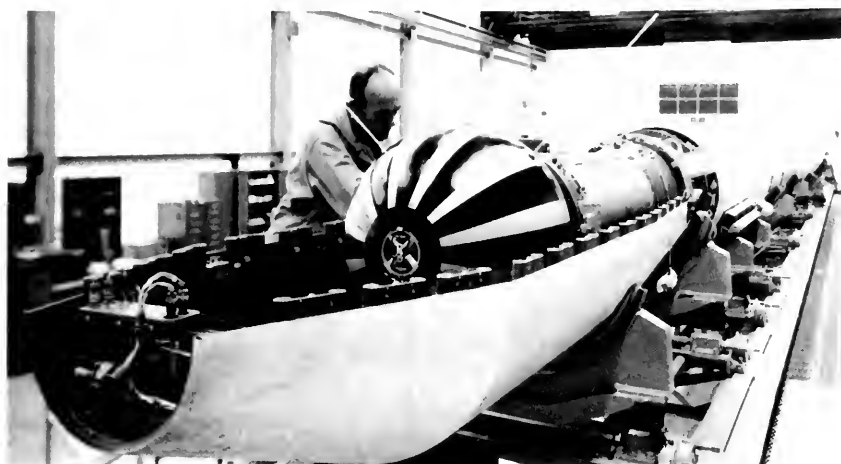
FIGURE A-42.—San Marco 1 being mated to Scout.
